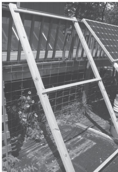
Wooden deck-mounted racking awaiting new panels
