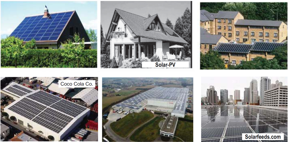
Fig. 5.4 – Six solar rooftops of residential, commercial and industrial installations
