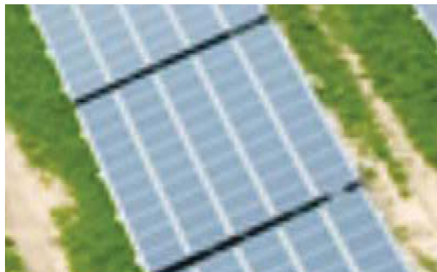
Fig. 8.4 – Multiple Solar Panel Mounts
